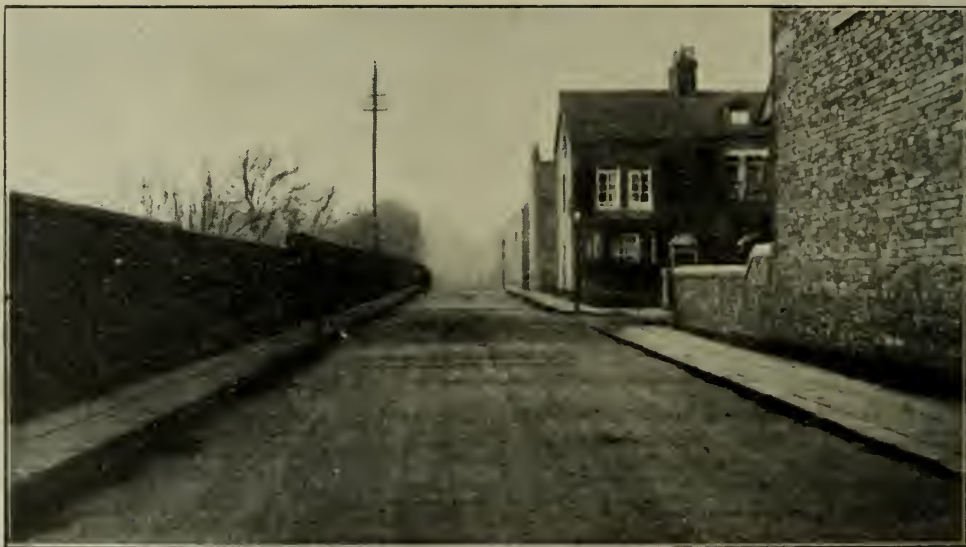
CONCRETE ROAD AT MIDDLESBROUGH.
